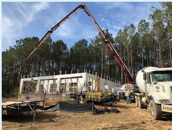
Figure 8. A FORTIFIED Home during construction in Fairhope, Alabama.
